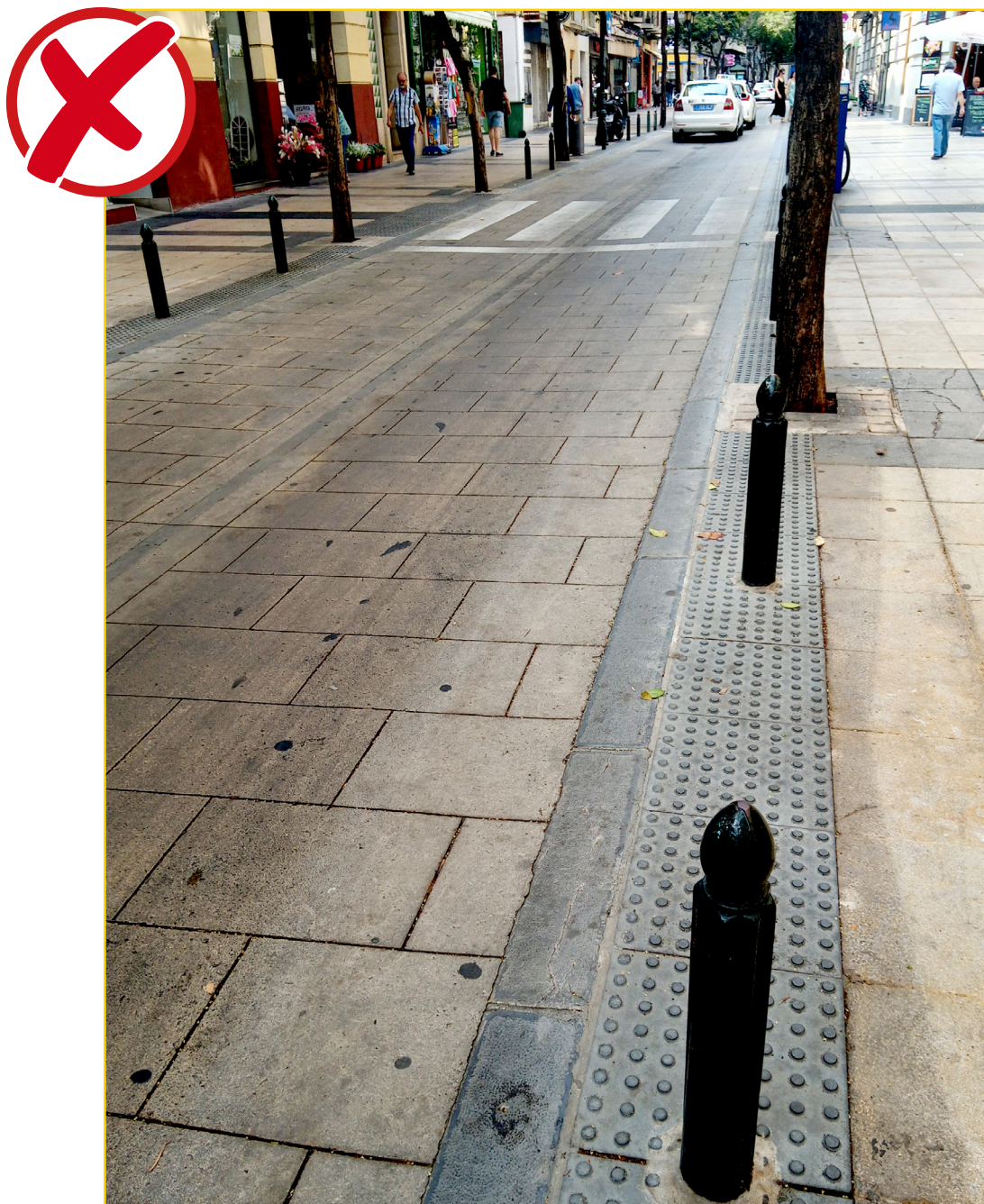
Image 35. There is no difference between the paving on the road and on the pavement.
