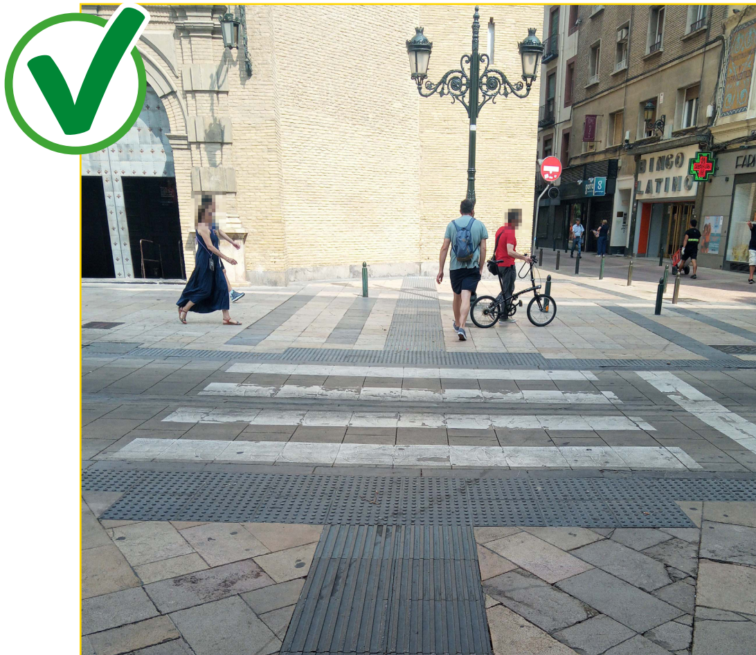
Image 38. Properly aligned guidance paving.
