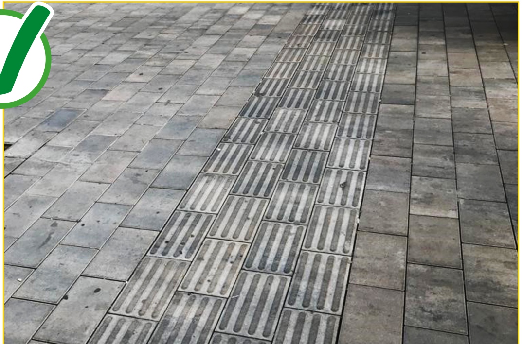
Image 16. Proper contrast in textures between the delineator and the adjacent paving.
