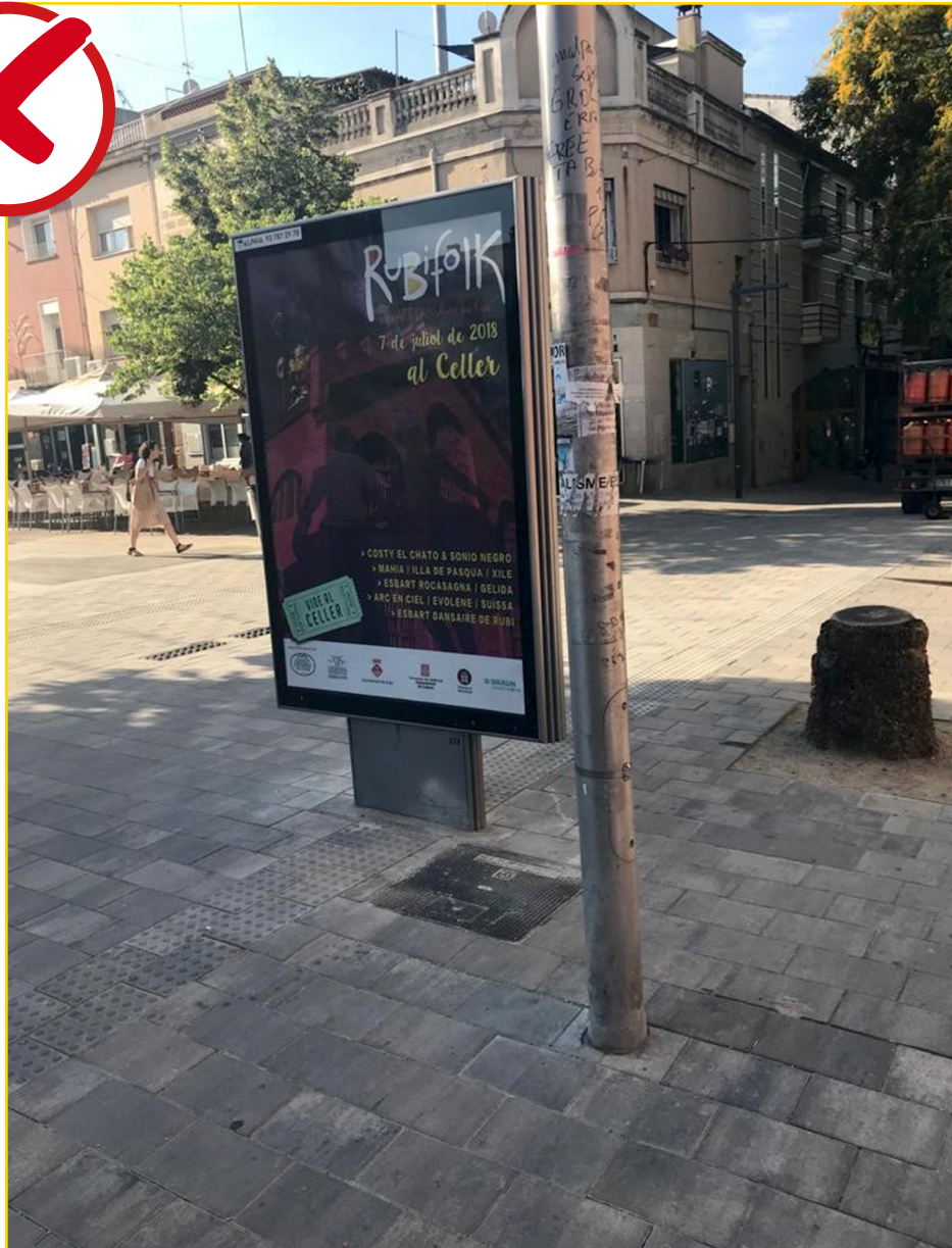
Image 17. Street furniture on visual tactile paving.
