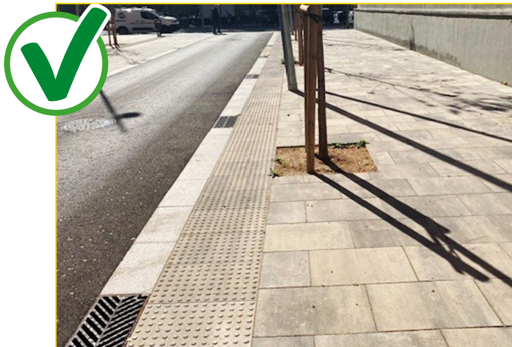
Image 33. Proper demarcation of pavement and road.
