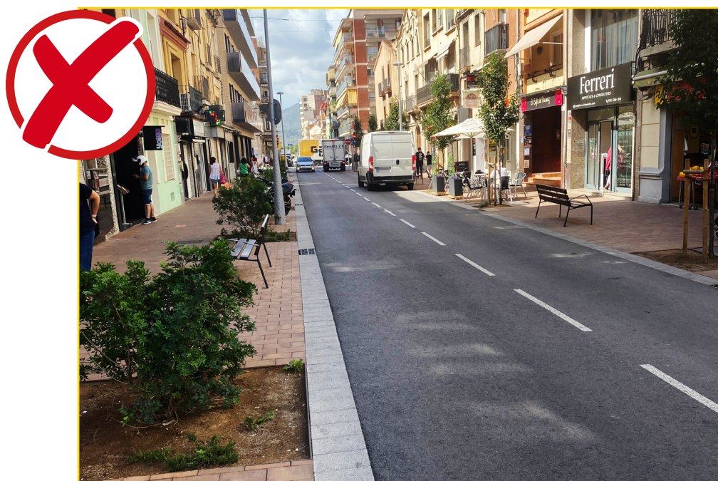
Image 34. Lack of demarcation through warning paving.
