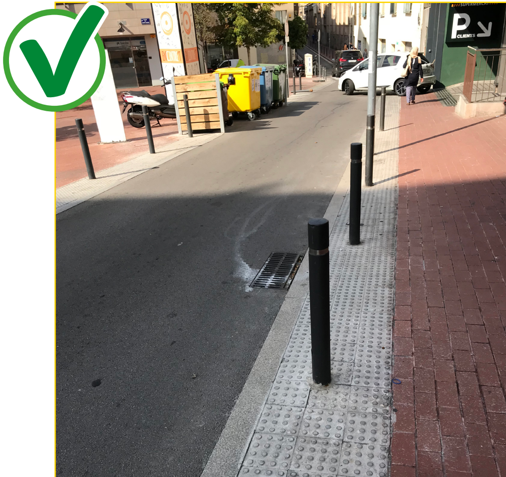
Image 30. Vehicular and pedestrian areas are clearly distinguishable.
