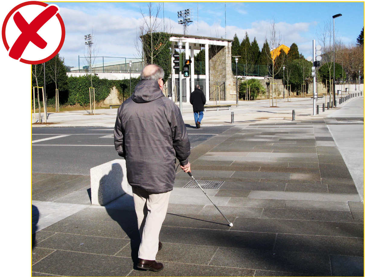
Image 36. Lack of markings.
