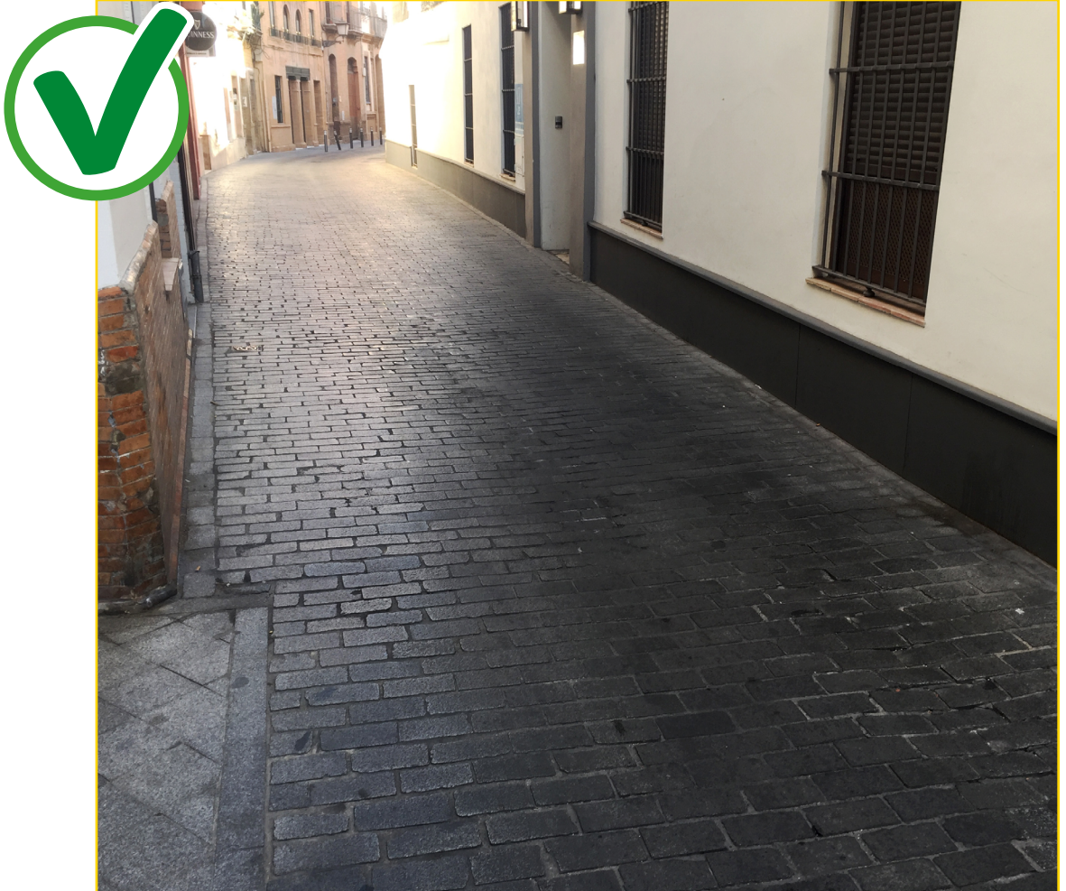
Image 21. Street where it is impossible to delimit a safe zone.
