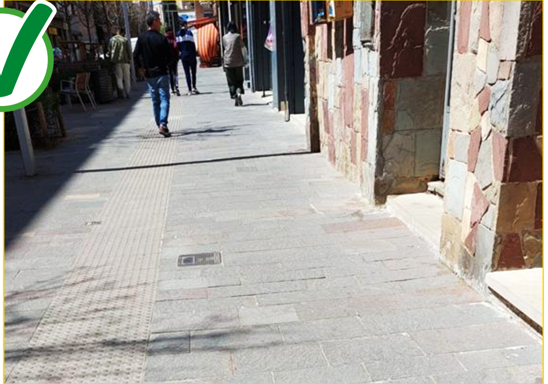
Image 15. Proper contrast in textures between the warning paving and the adjacent paving.
