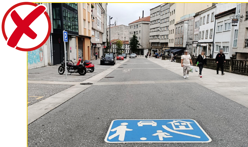
Image 39. Poor signage in a space with segregated traffic, suggesting that this space is for shared use.
