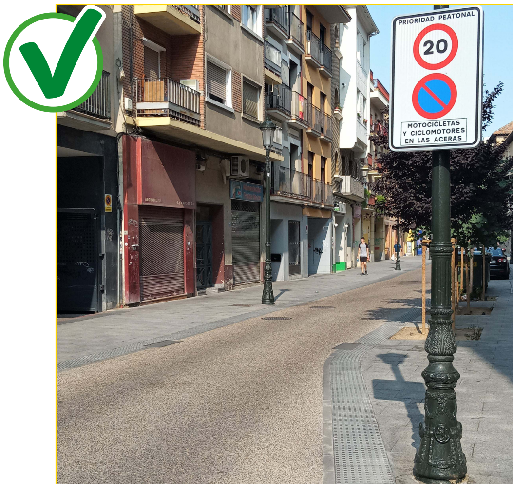
Image 40. Suitable signage providing information on traffic restrictions. However, there is not enough delimiting furniture alongside the visual tactile paving.
