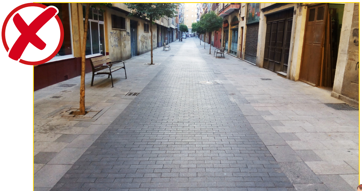
Image 10. Paving markings that suggest that vehicles have priority.
